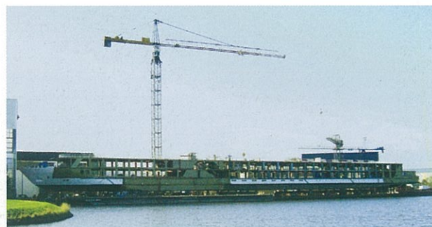
Amadeus Silver under construction at the Foxhol yard
